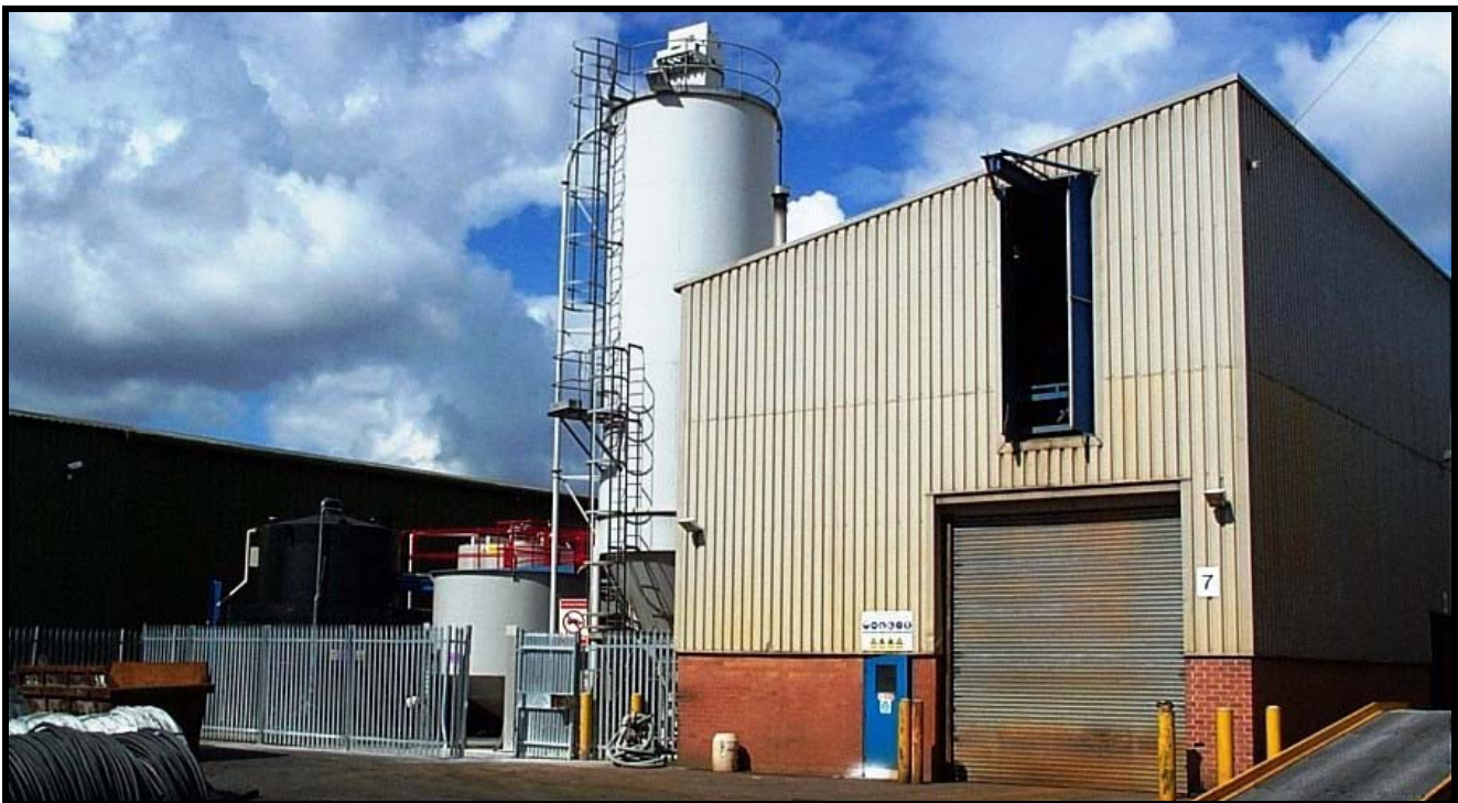
Main Effluent Treatment Plant Building
